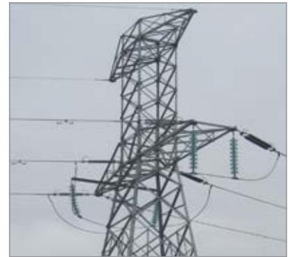
A 3-phase 110 kV transmission line carried on a steel pylon. The conductor carrying each phase is suspended from an insulator. The two conductors at the top of the pylon are connected to earth and act as lightning conductors.
