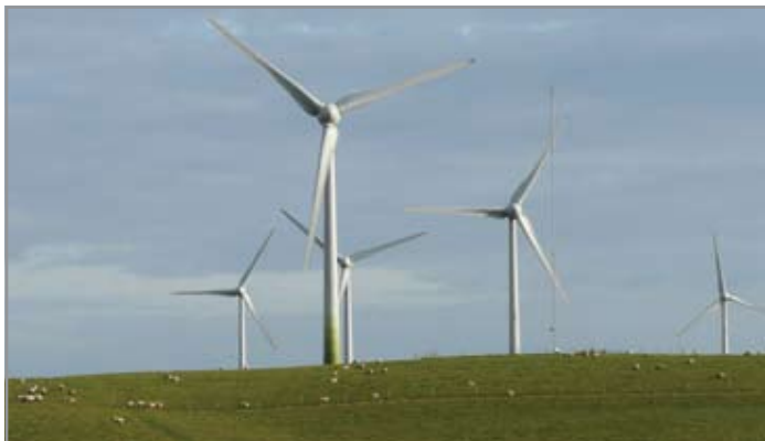
Fig. 1 Wind turbine generators
